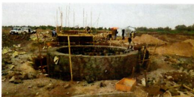
Slow sand filter water supply scheme under construction
